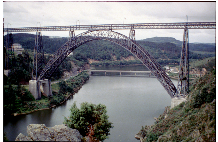
Garabit Viaduct - Eiffel
