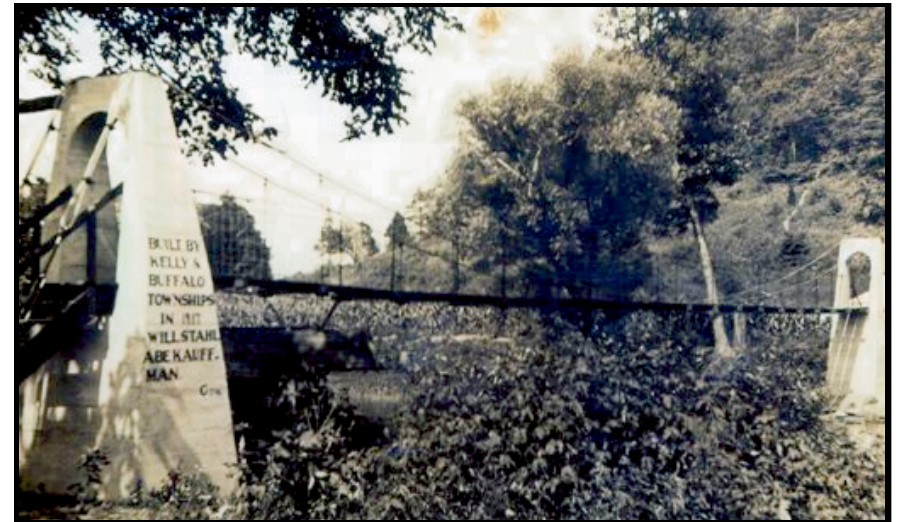
Buffalo Creek Bridge (1917)
