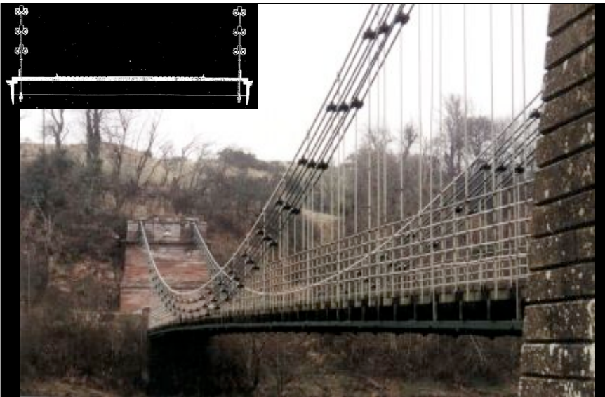
Union Bridge (1820) Samuel Brown
