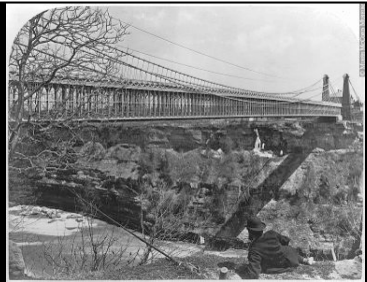
Niagara Railroad Bridge (1849) John A. Roebling
