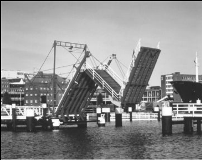
Fig. 16: Folding Bridge, Kiel, completed 1998
