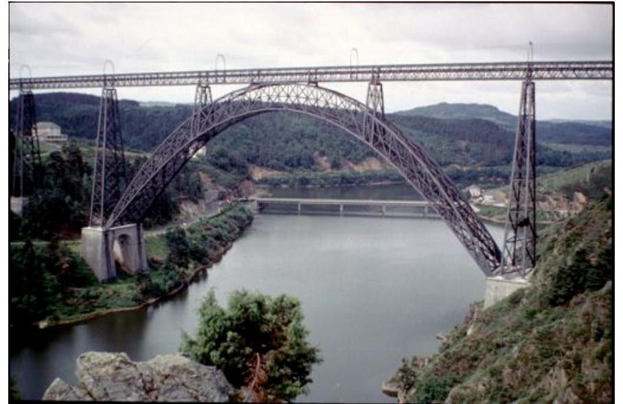
Garabit Viaduct - Eiffel
