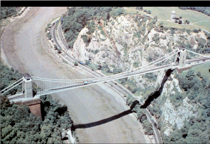
Clifton Bridge - I.K. Brunel - 1864 - 702 ft (vs 580 ft for Menai)
