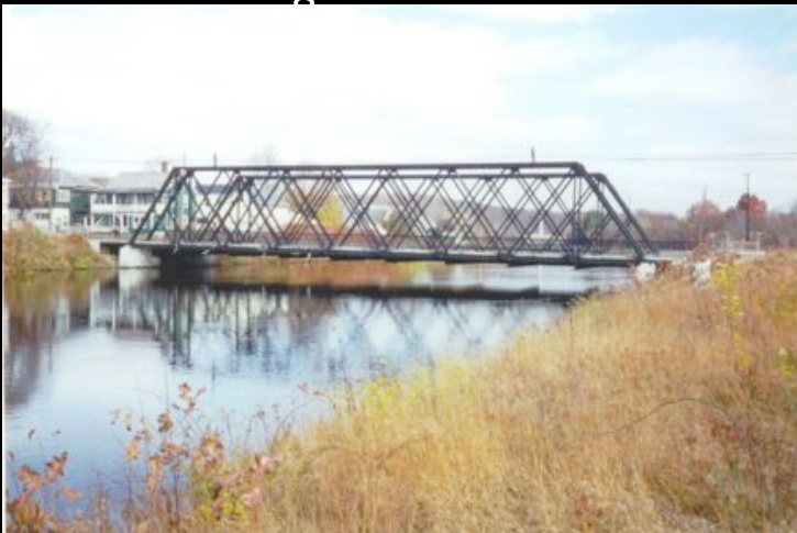
11 th Street Bridge – Double Intersecting Warren Truss 1915
