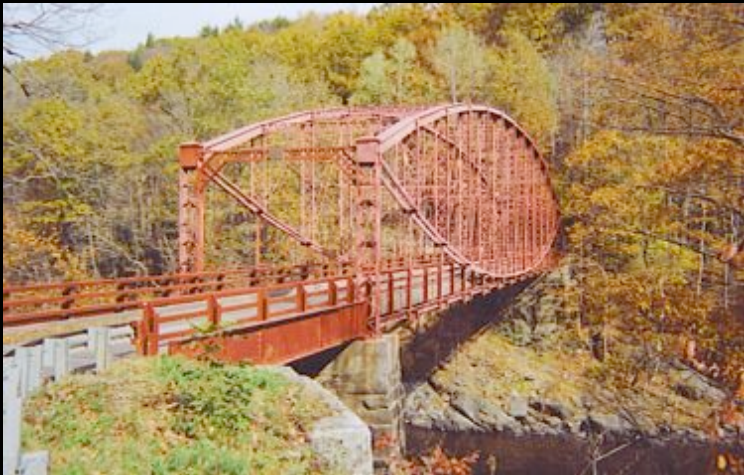
Bardwell's Ferry Bridge, Shelburne, Ma.
