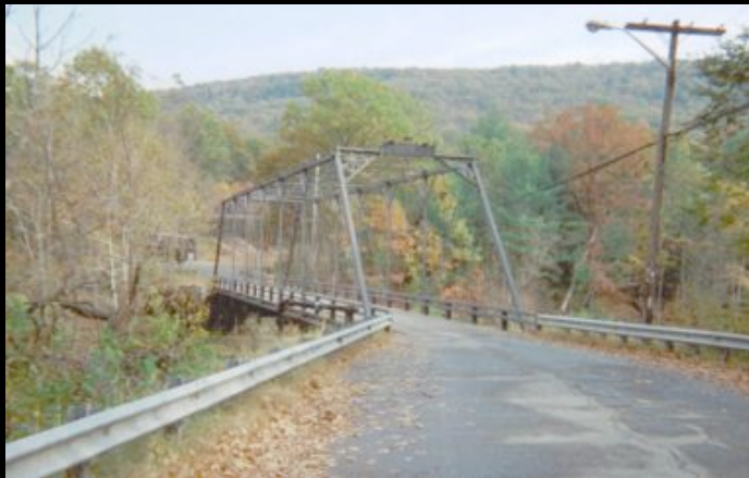
Farley Rd. Bridge – Erving (Phoenix Bridge Co.)
