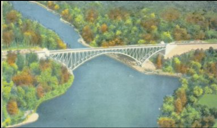
French King Bridge – Irving Steel Deck Arch Bridge 1932
