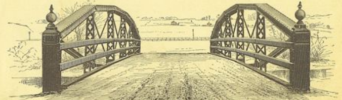
BRIDGE AT JAMESTOWN, CHAUTAQUA COUNTY, N. Y. Span, 70 feet. Roadway, 10 feet wide.
