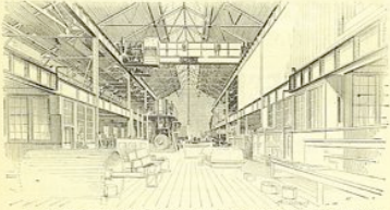
The above illustration is taken direct from a photograph and shows the interior of a Forge Shop designed and built by us for the West. Coast & Great Ship and Engine Building Co., at Philadelphia, Pa. The Forge Shop is 33 ft. in width and 50 ft. in length, the adjacent Boiler Shop covers on the right being 25 ft. in width and 50 ft. in length. The Smith Shop is controlled by a Travelling Crane as shown. The building is covered with Corrugated Iron.
