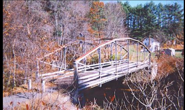
Depot Rd. Bridge, Colchester, N.H.
