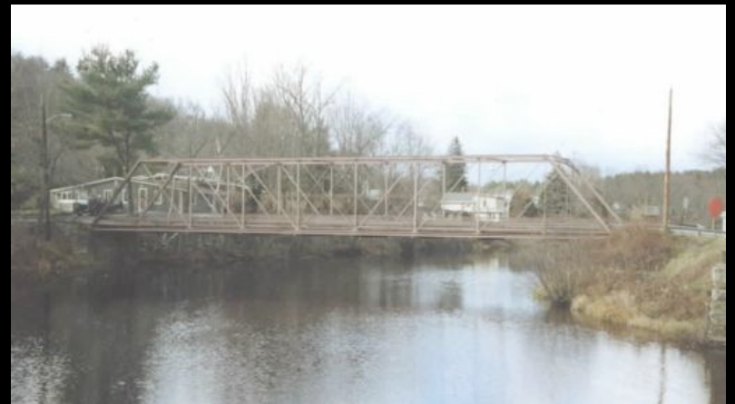
Hotel Street Bridge – Florence
