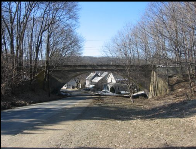
1 st Avenue Bridge – Turner's Falls
