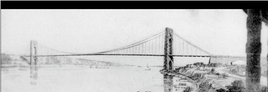
George Washington Bridge - Othmar Ammann - 3500 feet - 1931
