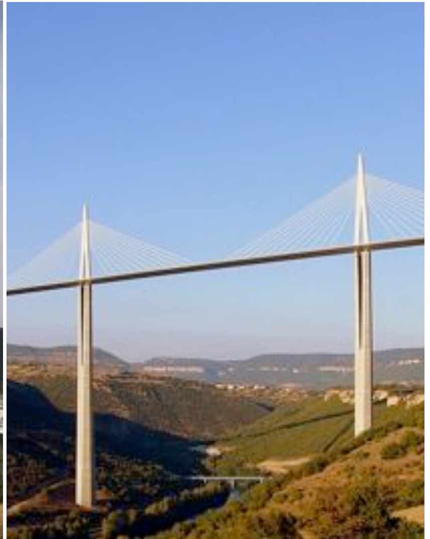
2004 Milau Viaduct by M. Virogleux
