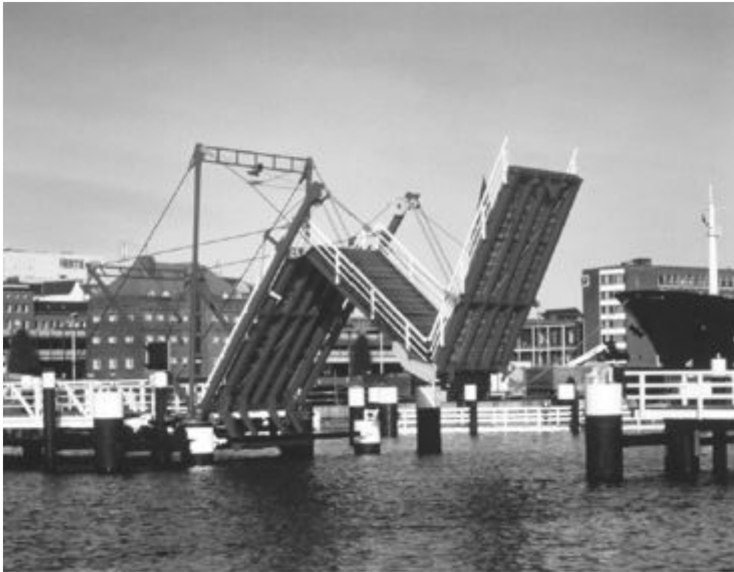
Fig. 16: Folding Bridge, Kiel, completed 1998
