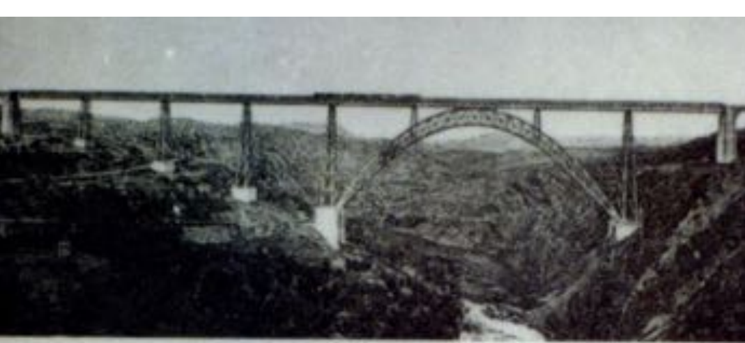
PONT DE GARABIT Designed by Eiffel the engineer.
