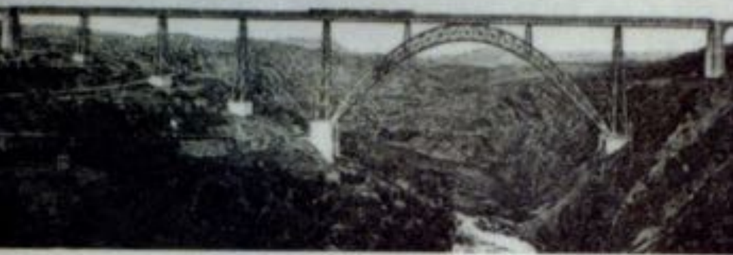
PONT DE GARABIT Designed by Eiffel the engineer.
